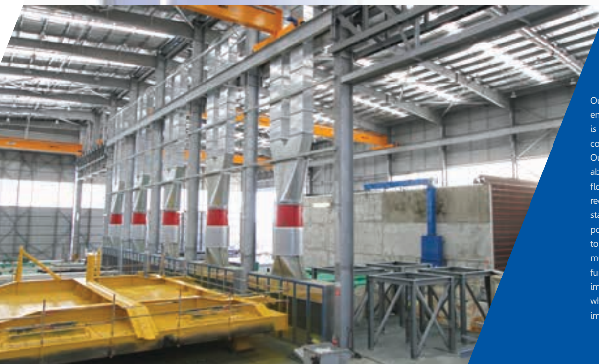
Specialist welding of super duplex LNG piping.
