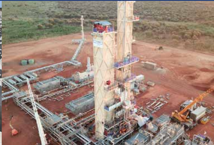
STRUCTURAL, MECHANICAL AND PIPING
